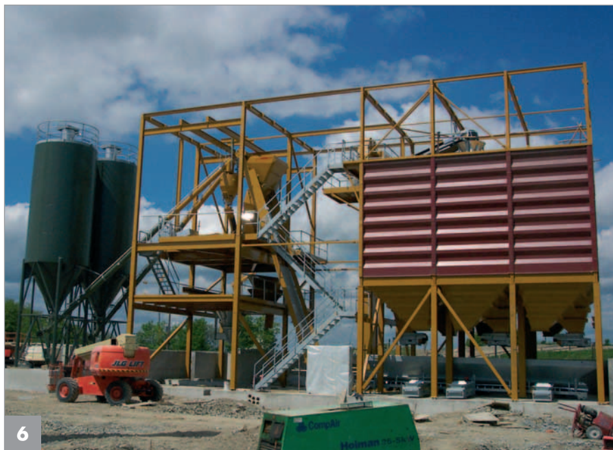
Batching plant without cladding
