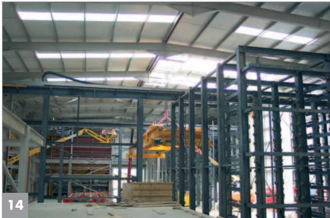
Curing chamber and rack operator during the assembly
