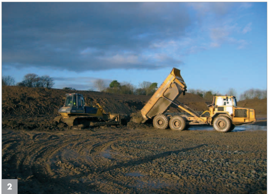
Soil composition of the building site
