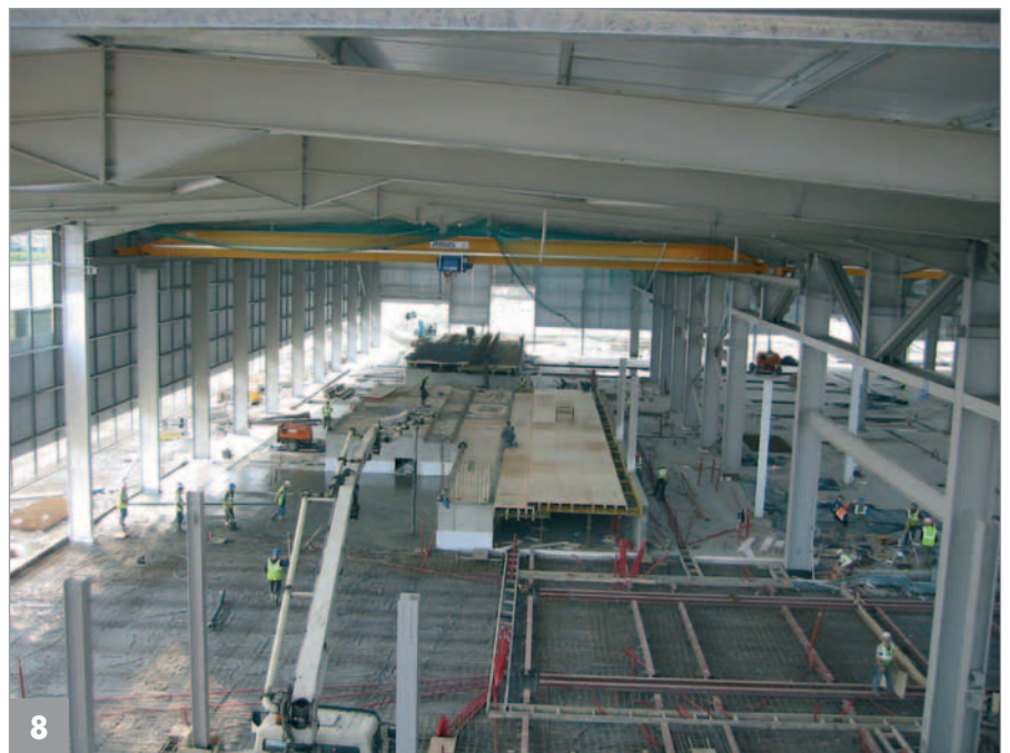
Demoulding area in the construction stage
