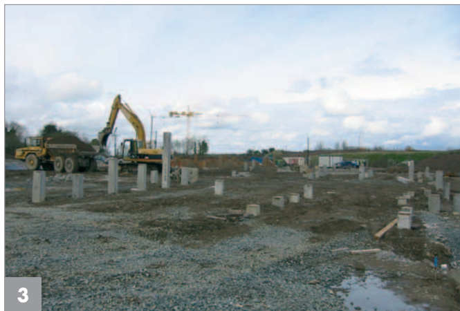
Piles in the area of the curing chamber
