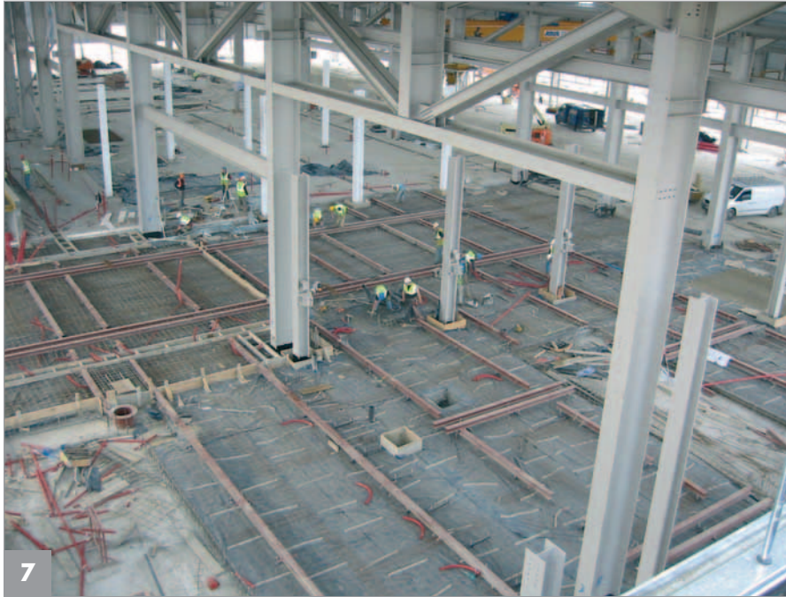
Preparation of the floor plate
