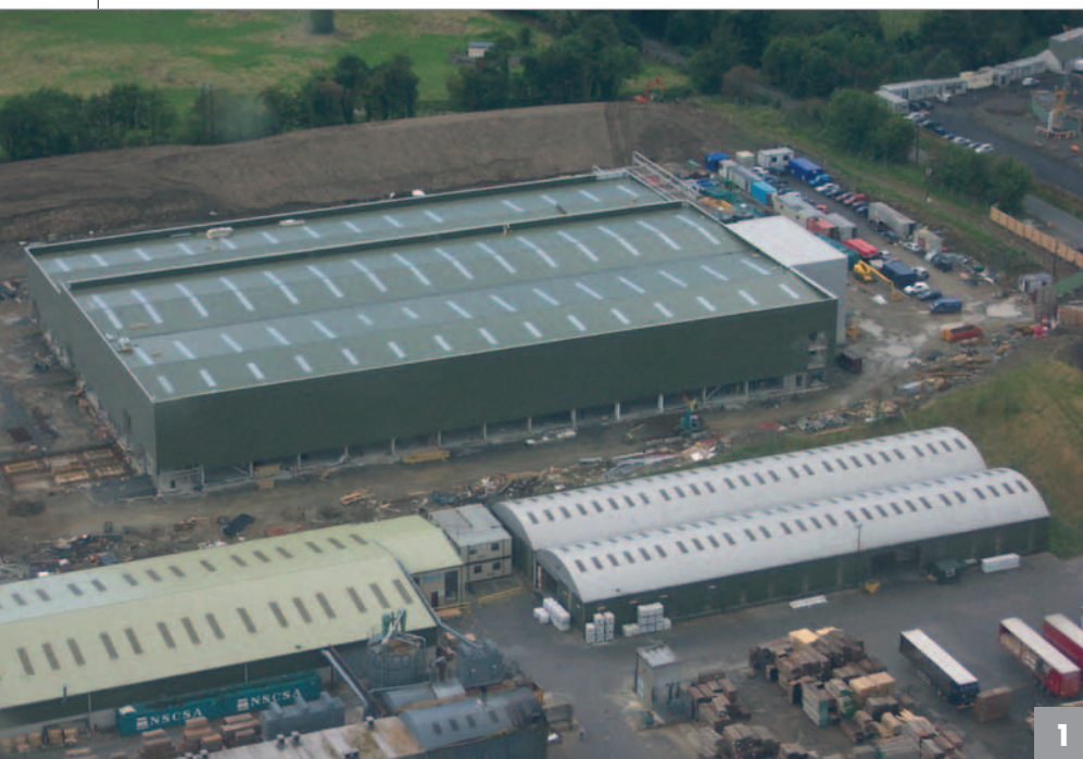
Factory building with three wings and batching plant
