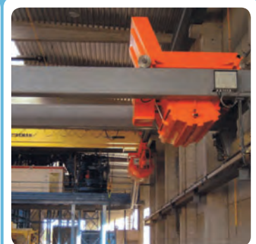
Rollover bucket and concrete distributor
