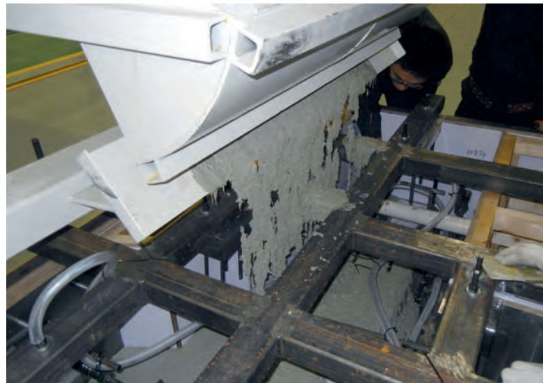
Concreting the first component
